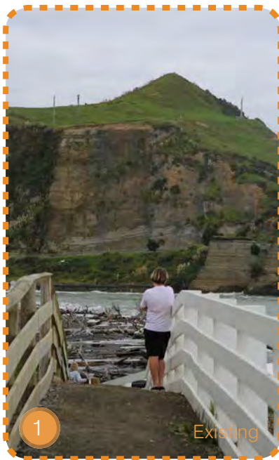
1 - Existing access to Mokau Spit which has been successful.
