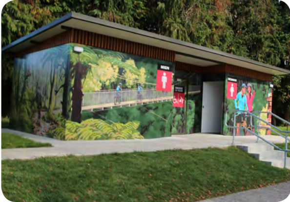
Distinctive toilet in Benneydale - an approach for a new toilet facility.
