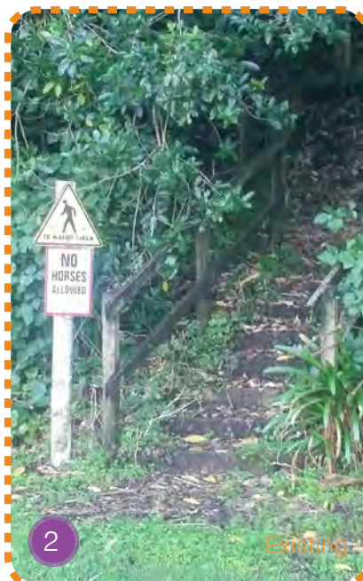
2 - Existing access to boat ramp which needs improvement.
